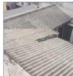
Coperture in amianto
